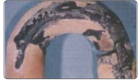
Fig. 4. Thermal Fatigue Failure in U-bend.
