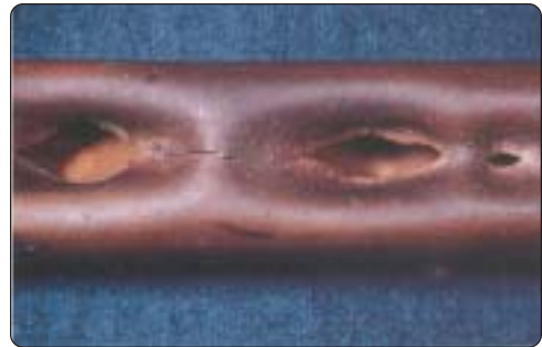
Fig. 2. Tube Damage from Steam Hammer.
